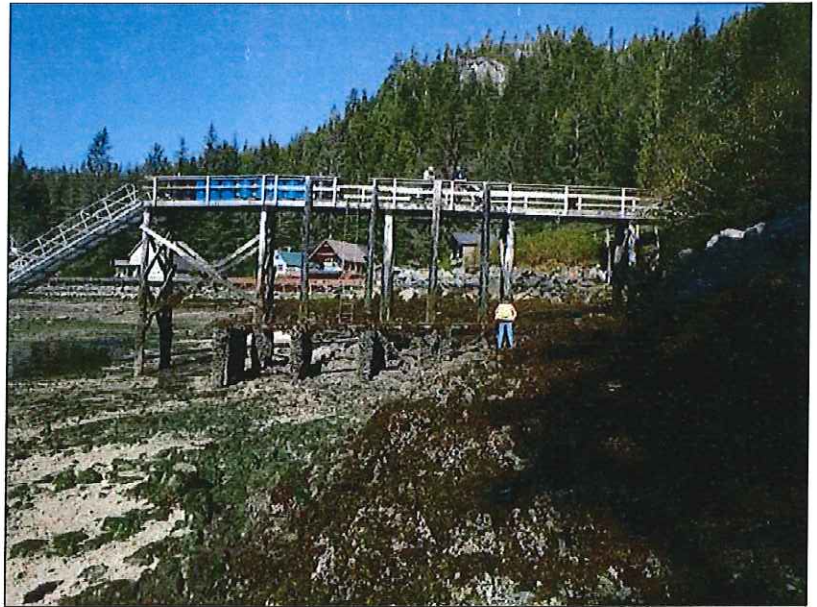
EXISTING TRESTLE AND BOAT GRID
